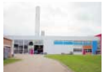
Dordrecht / NL - Home of the world's largest flowmeter calibration rig.
