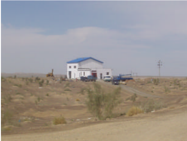
Pump station in the desert
