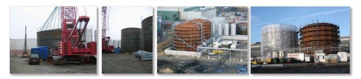
The installation of the big storage tanks took several weeks. Due to the salt-laden air the non-protected steel already corroded extremely. The blasting and external coating had to be carried out fast and accurately.
